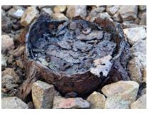
Hidden corrosion damage of the baseplate
